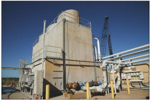
Testing of the walls showed corrosion rates between 16.72 and  $67.91\mu$ m/year, which indicates a low to moderate level of corrosion.
